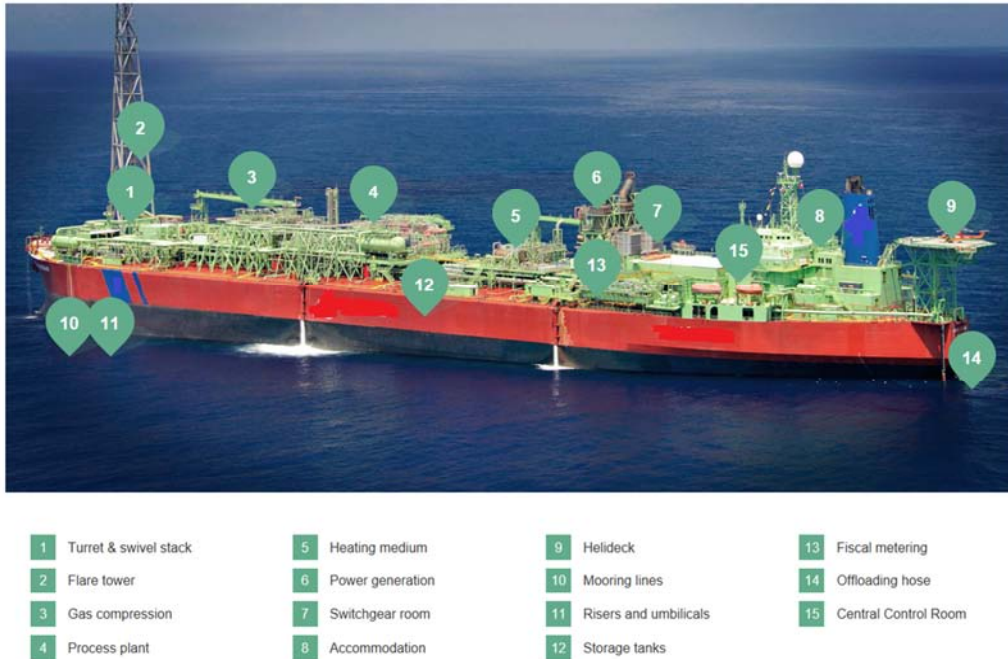
Figure 5. Main areas of the FPSO.
